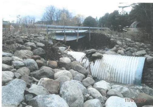
Damages to Yaw Road due to a 2019 storm event
