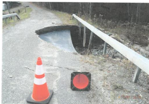
Damages to Yaw Road due to a 2019 storm event
